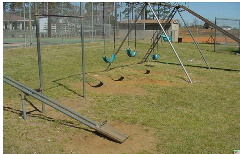
This playground doesn't use any protective surfacing in the event of a fall.
